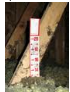
Insulation depth gauge– required every 300 square feet in attic
